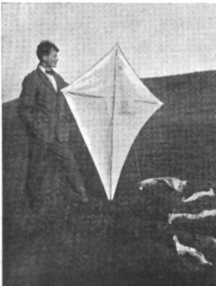
Kite used in successful experiments with portable aerial.
