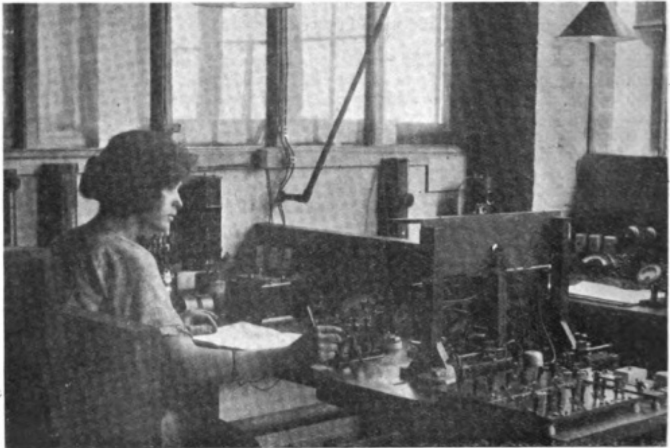
A Test Bench where Valves are examined and data recorded.
