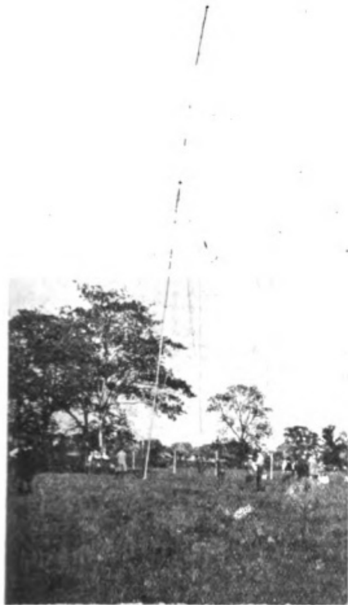
The mast nearing the vertical position.
