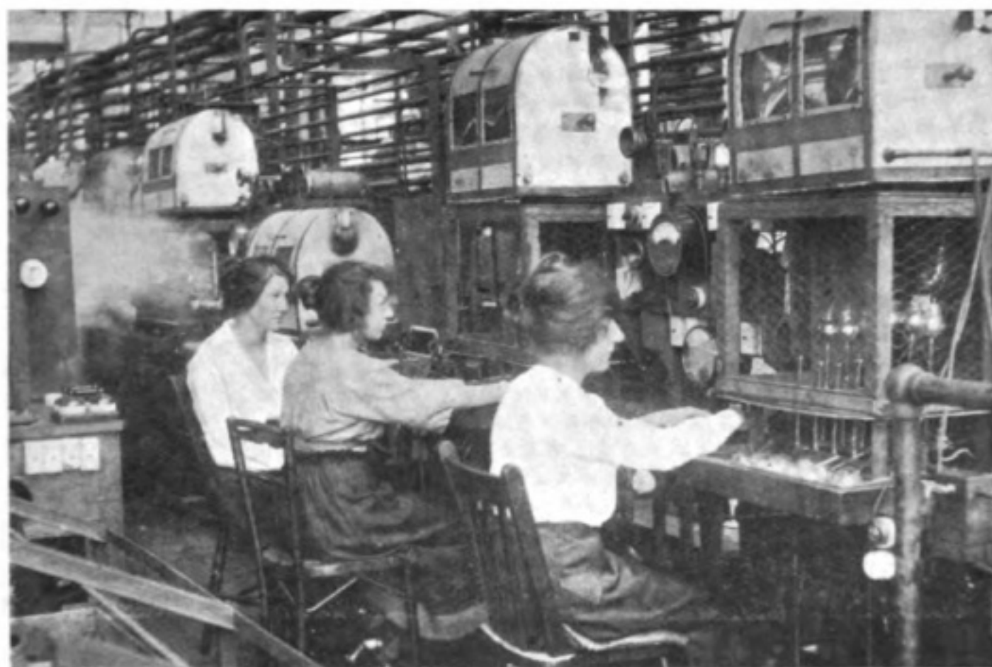
Valves of the "R" type connected to the pump whilst the operator controls the potentials applied to the electrodes.
