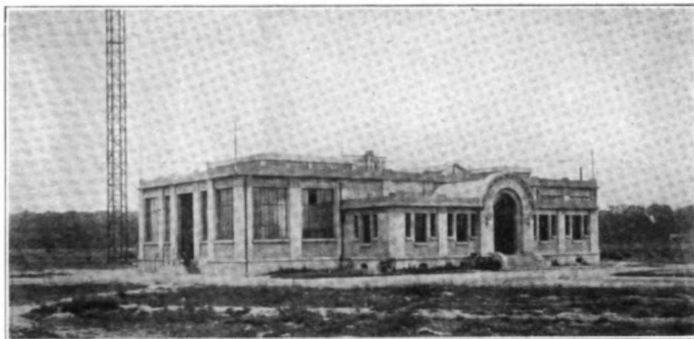
Fig. 1. The station building of the Continental transmitter.
